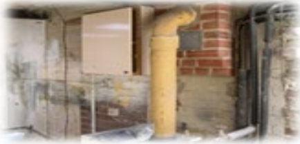
Asbestos Cement Boiler Flue
